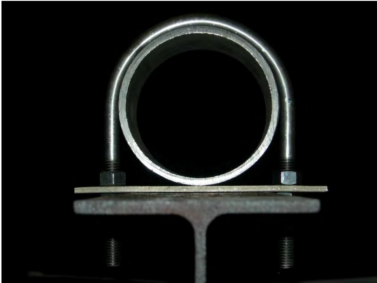
FIG. 14 U-BOLT WITH A BASE STRAP
