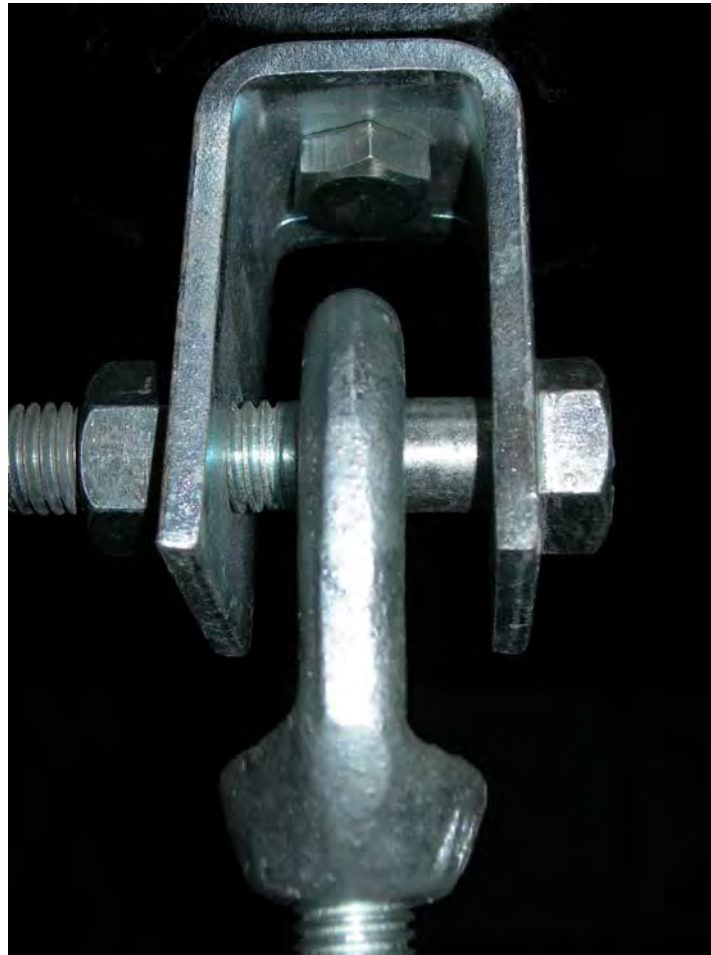
FIG. 36 EYE NUT ON A WELDED BEAD ATTACHMENT
